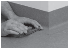
Cut out the floor covering that will be laid on top of the skirting
