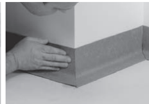
line. Lay HSLA skirtings. Press properly.
